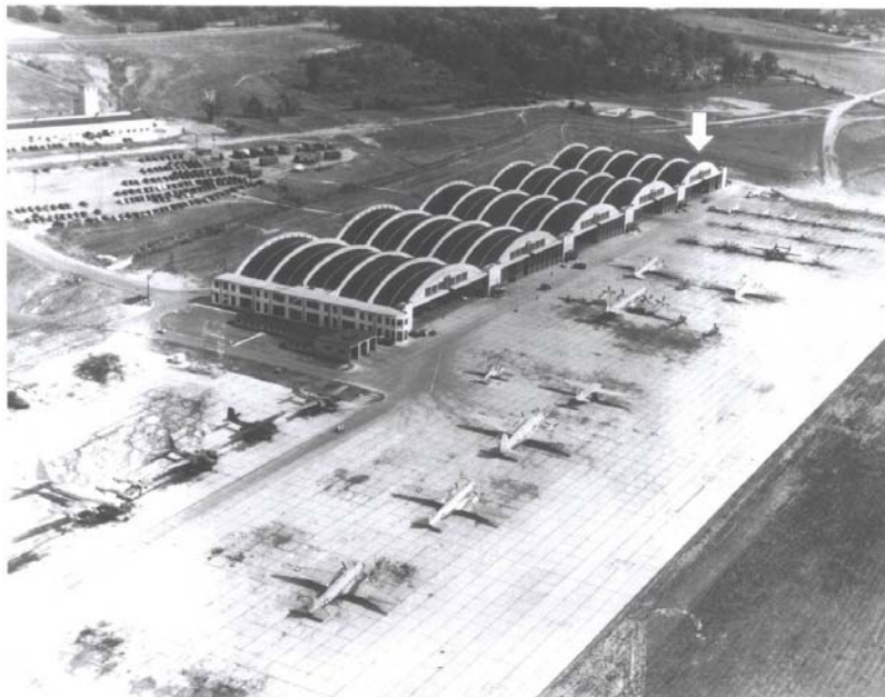
Hangar complex #4 at Wright Patterson AFB. Bay "E" is the furthest hangar to the right indicated by the arrow.
